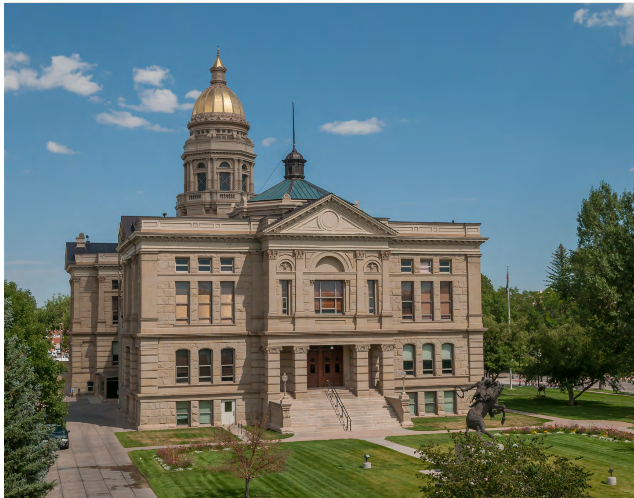
Figure 2.1: Exterior View looking East
