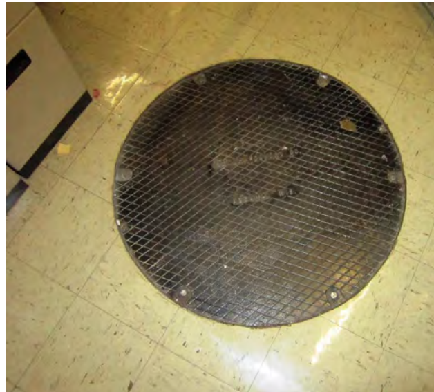
Figure N.01.07 - Existing Watertight Cover over Interior Well, Room B7
