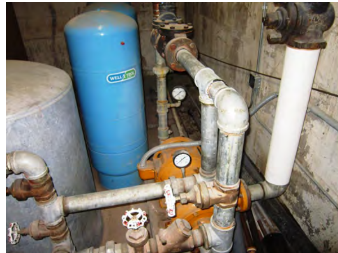
Figure N.01.08 - Existing Well Pump & Buffer Tanks, Water Svc Rm, Central Utility Plant
