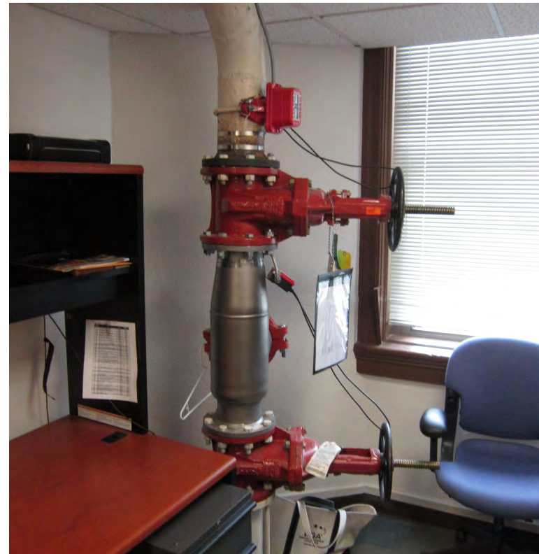
Figure N.02.03 - 6" Fire Protection Water Service with BFP, Capitol Bldg Basement
