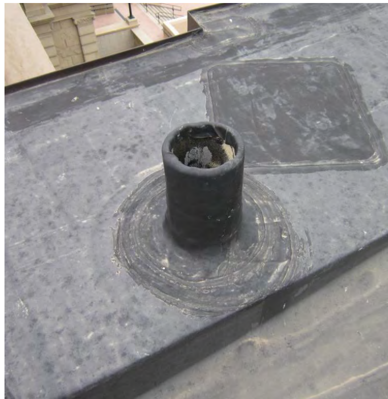
Figure N.02.04 - Existing Sanitary Vent Penetration of Roof
