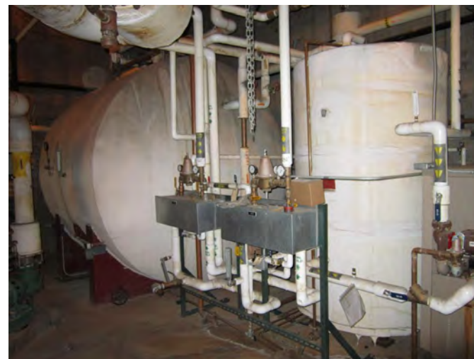
Figure N.01.10 - 10,000 Gal Solar Domestic Water Storage Tank, Herschler Basement MER
