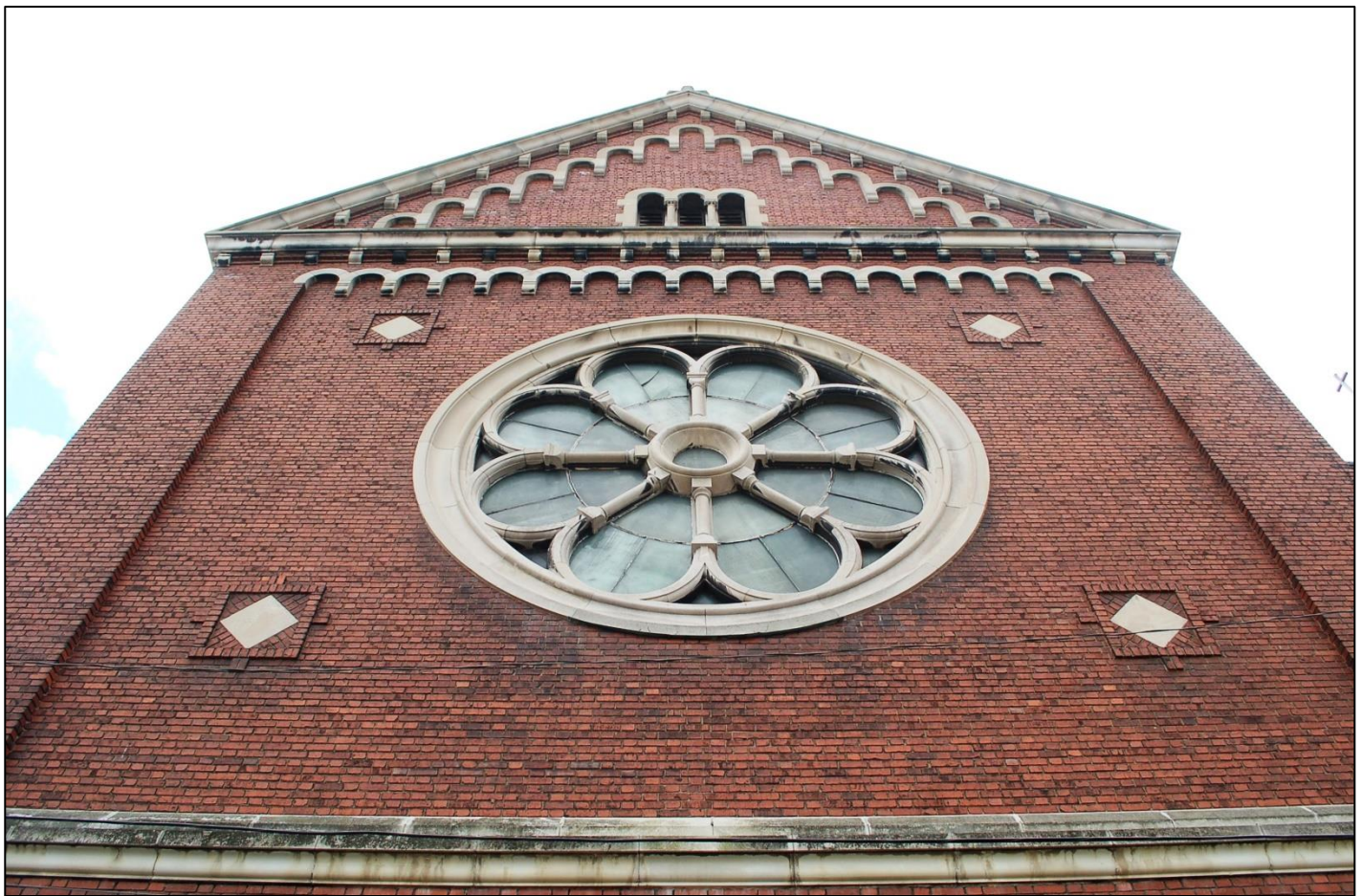
Photo 9: 823 Climax Street, Rose Window, Northern Transept, March 2016.
