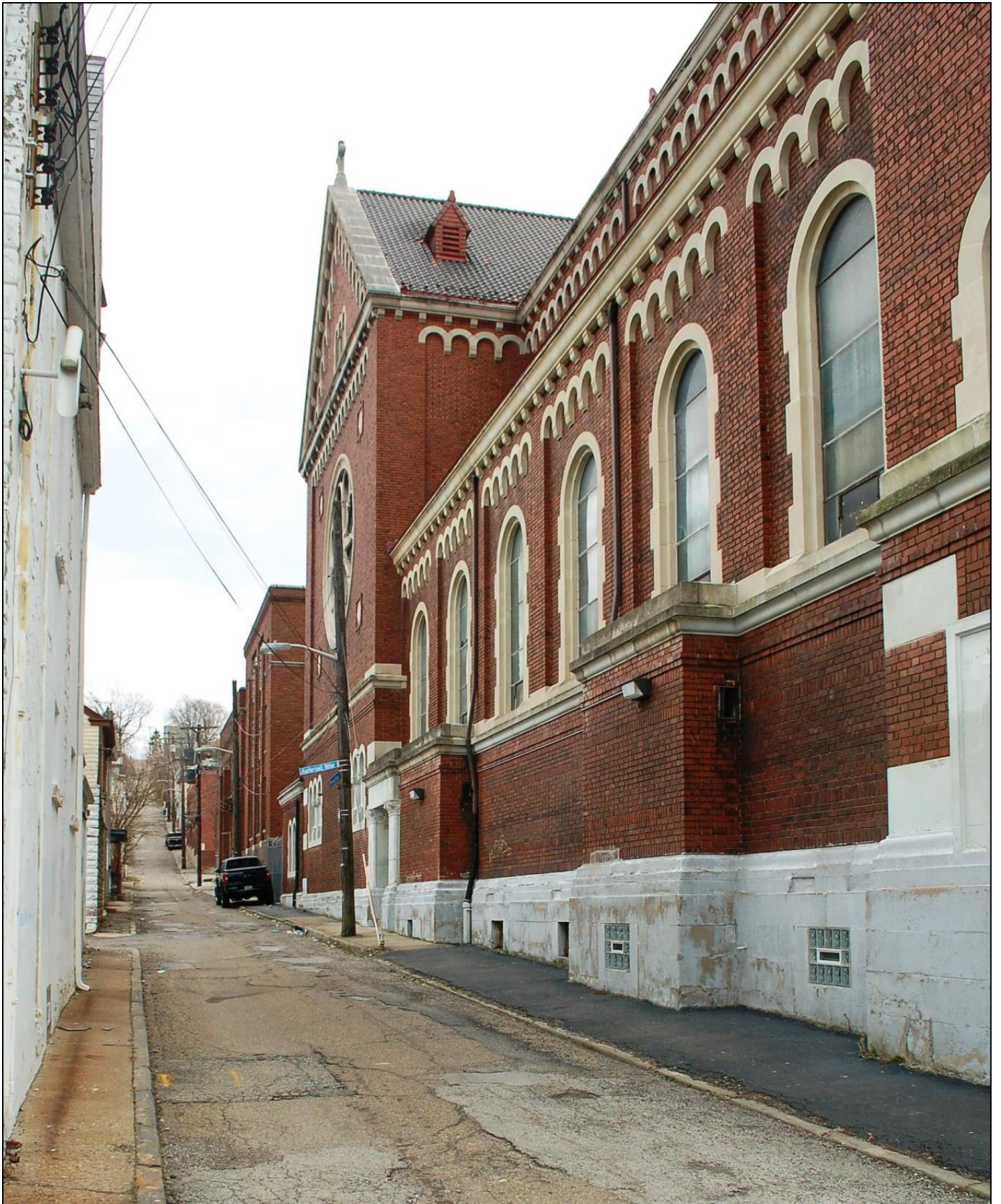
Photo 4: 823 Climax Street, Northern Elevation Looking East on Proctor Way, March 2016.
