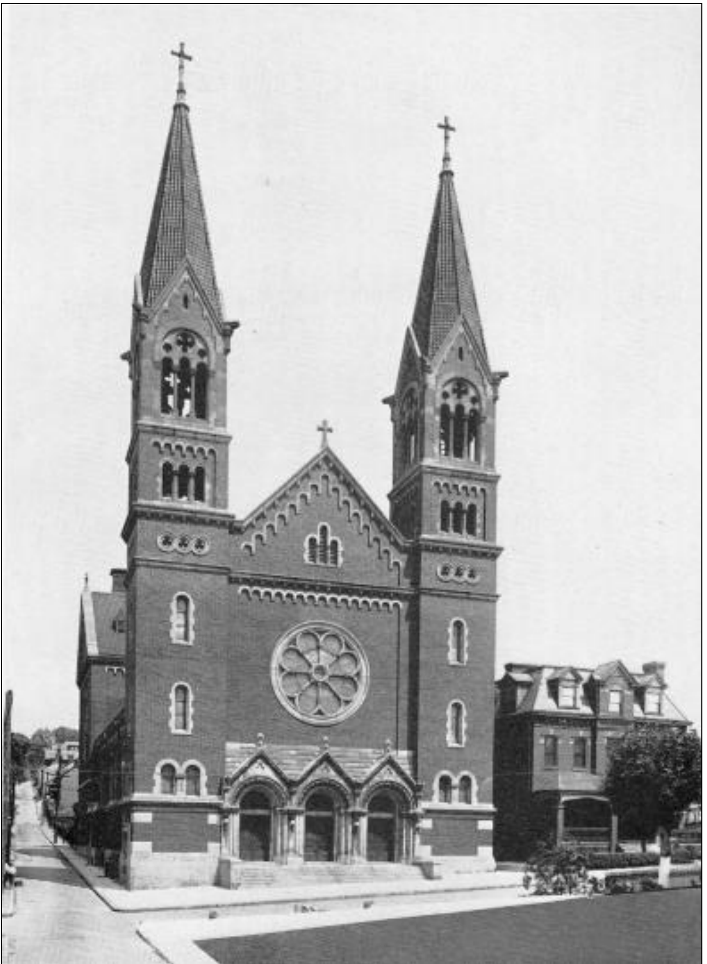
Photo 1: 823 Climax Street (then St. George Roman Catholic Church) and Parish House (now demolished), c. 1938.
