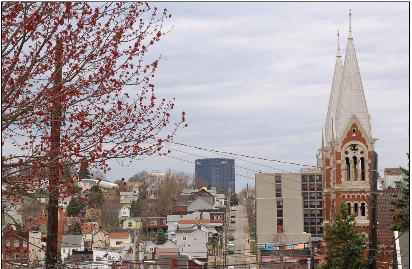
Photo 3: Spires of 823 Climax Street, looking North toward Downtown Pittsburgh, March 2016.
