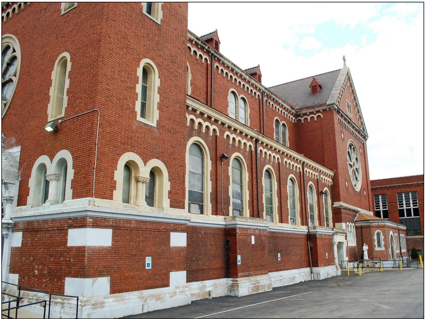
Photo 5: 823 Climax Street, Southern Elevation Looking East, March 2016.
