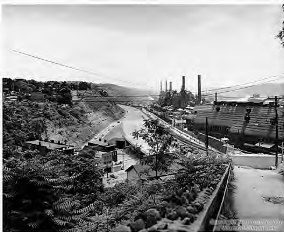
Fig. 8. Shrader, John. Penn-Lincoln Parkway East Bates Street Construction . 1956. Allegheny Conference on Community Development Photographs. Accessed: https://historicpittsburgh.org/islandora/object/pitt%3AMSP285.B010.F30.I04
