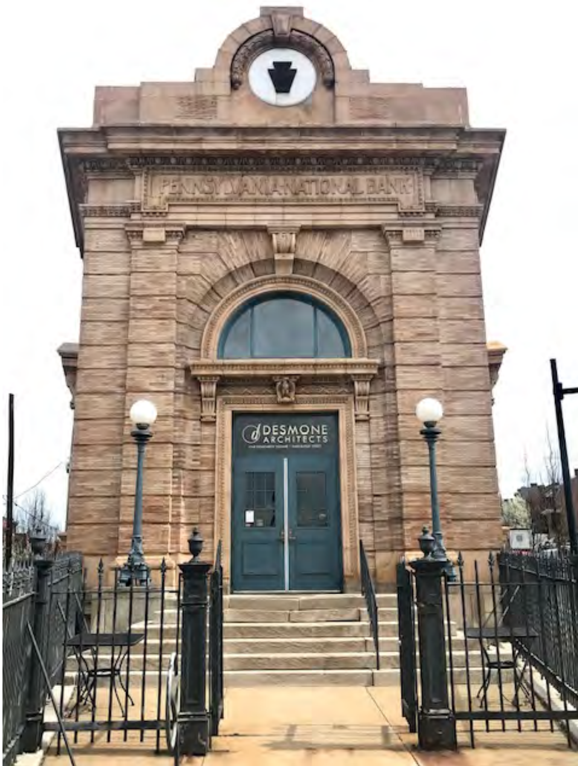
Photo. 3. Former Pennsylvania National Bank Building, Primary Façade, August 2019. Source: Matthew W.C. Falcone.
