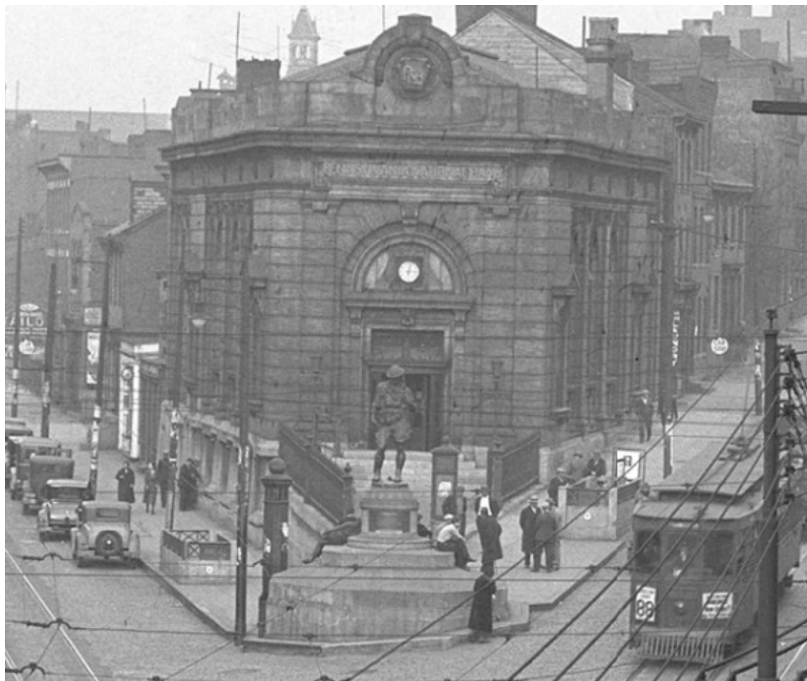
Figure 6 (detail). Pennsylvania National Bank Building, Detail . 1932. Pittsburgh City Photographer. Accessed: https://historicpittsburgh.org/islandora/object/pitt%3A715.3217591.CP
