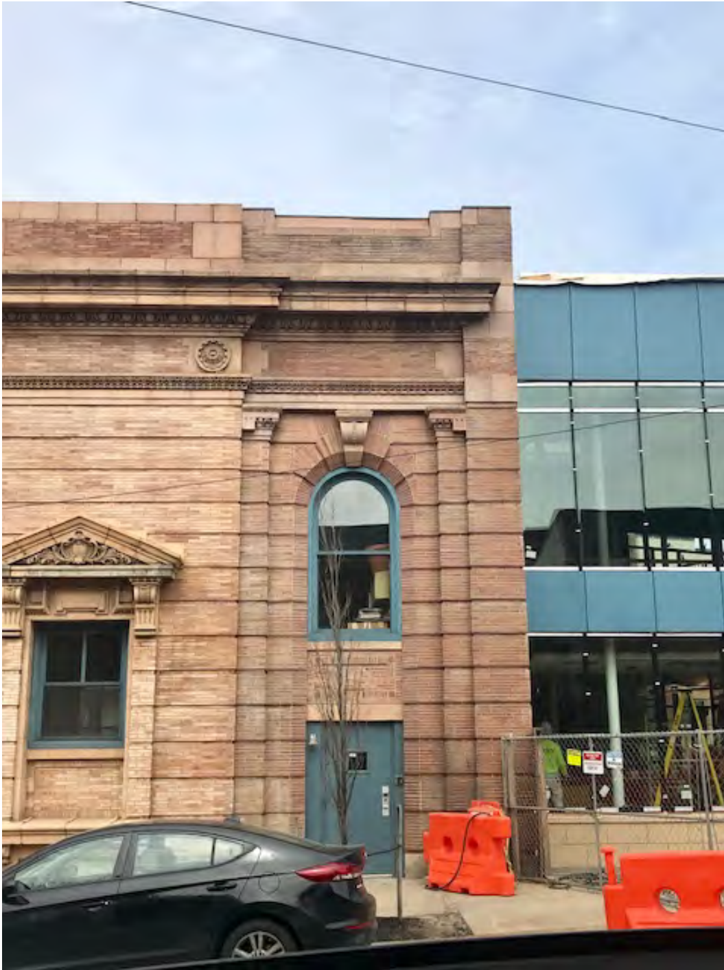
Photo. 11. Former Pennsylvania National Bank Building, Penn Ave. Addition, April 2019. Source: Matthew W.C. Falcone.
