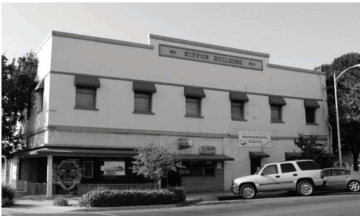
The Nippon Building on the northwest corner of Kern and F Streets, former home of the Rex and Cal theaters. 2013.
