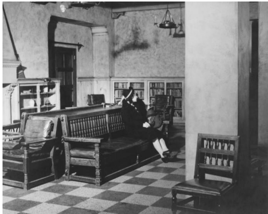
Figure 22: Lobby of 331 East 70 th Street
