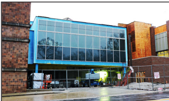
Washington University athletic center in progress.
