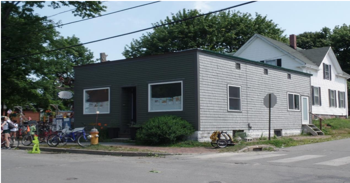
115 Island Avenue, c1904 New England Telephone Co., Telephone Exchange
