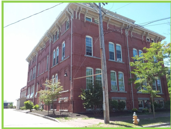
Shailer School 56-60 North Street (1882) Proposed Landmark located within the boundary of the historic district.
