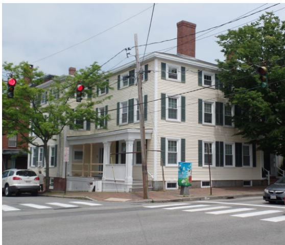
Federal-style 235 Cumberland Ave. in Bayside
