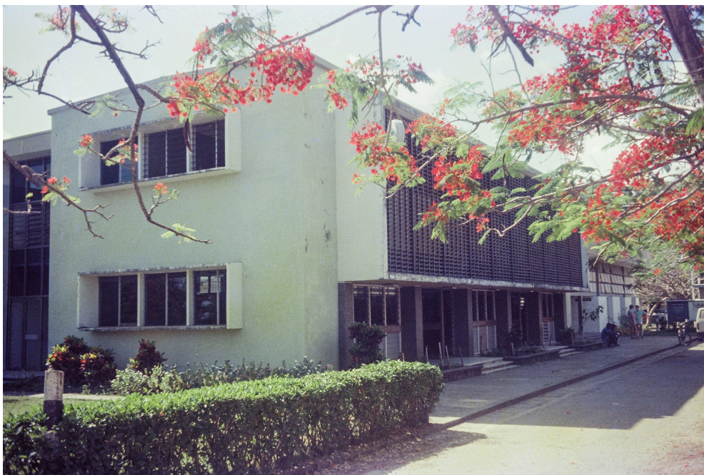
Fig 4. General Post Office, Honiara, 1970s. Photograph by Ann Stevenson.
