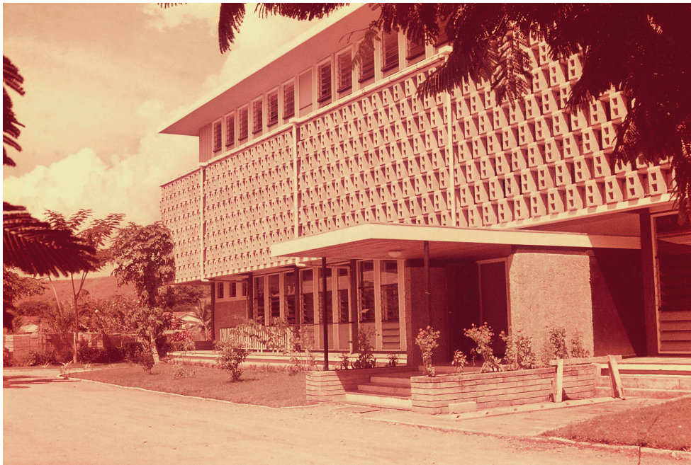
Fig 1. The Public Works Department Building, 1962. Photograph by Charles Stevenson.
