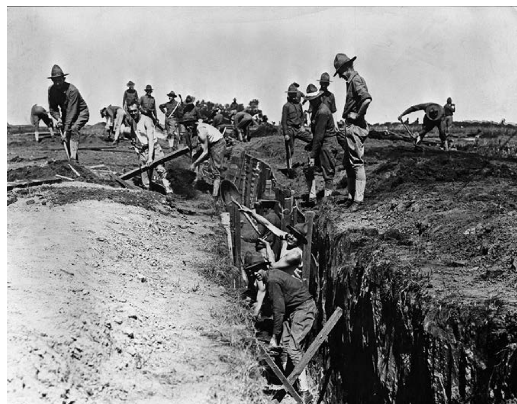
Americans troops at Fort Snelling training in the construction of trenches
