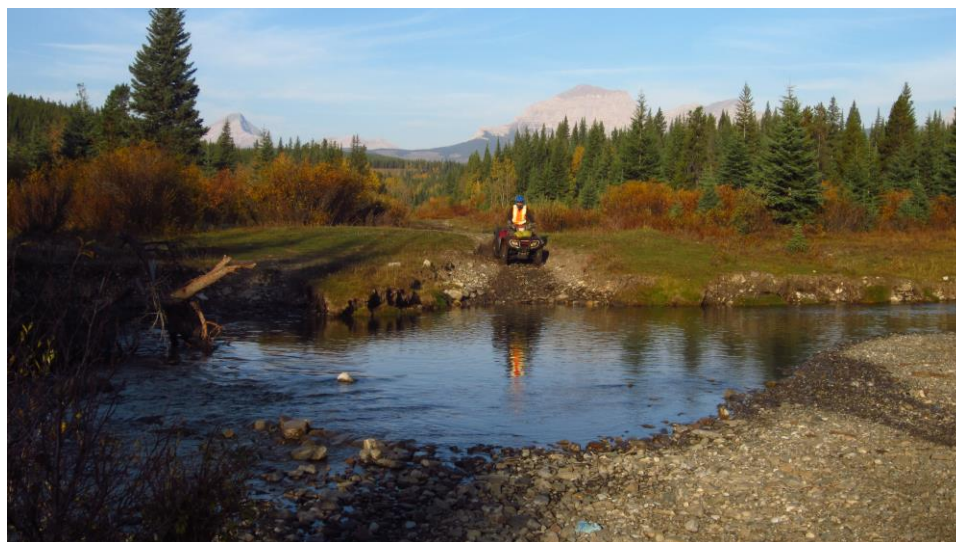
Plate 5. Photograph of an unregulated ford crossing at a large permanent stream showing widened bank widths at the crossing.
