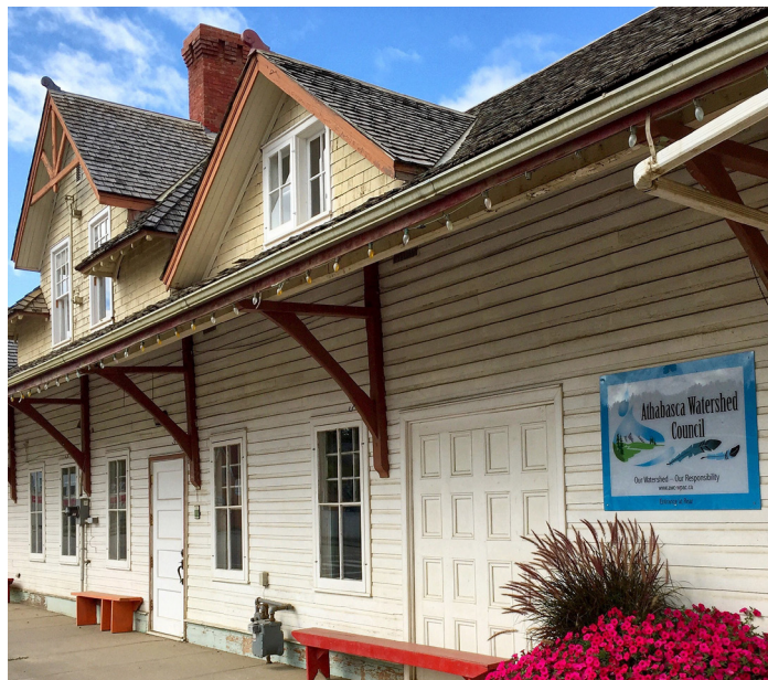
AWC's new office location - in the Athabasca Train Station.
