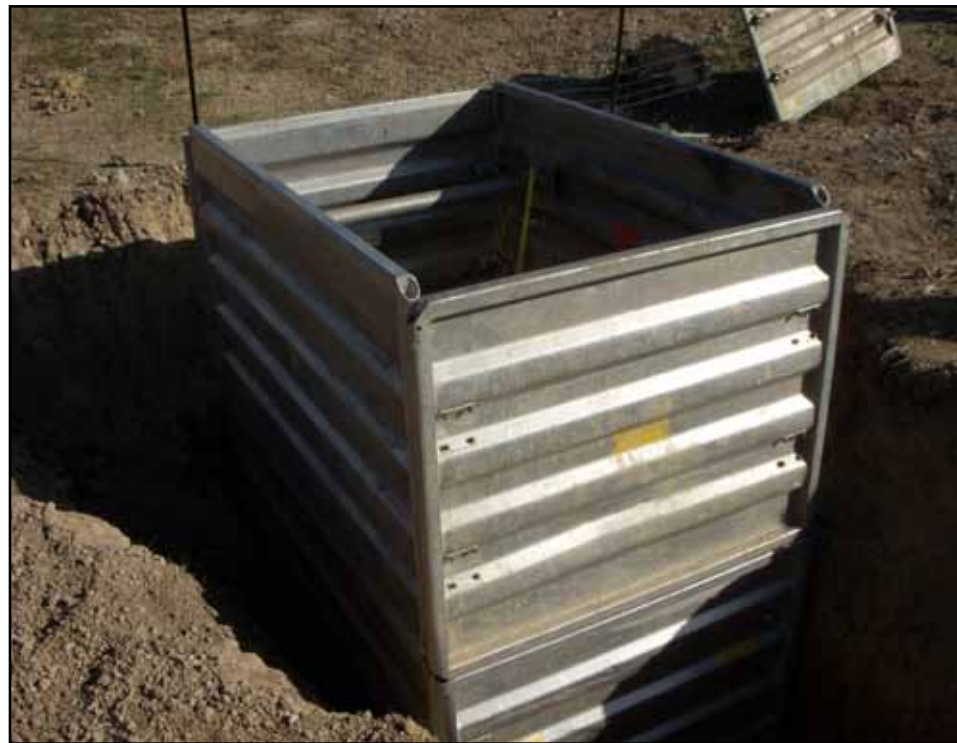
Four-sided shoring is now the norm for repair and maintenance.
