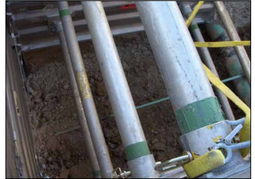
Miller Pipeline in a welding pit.
