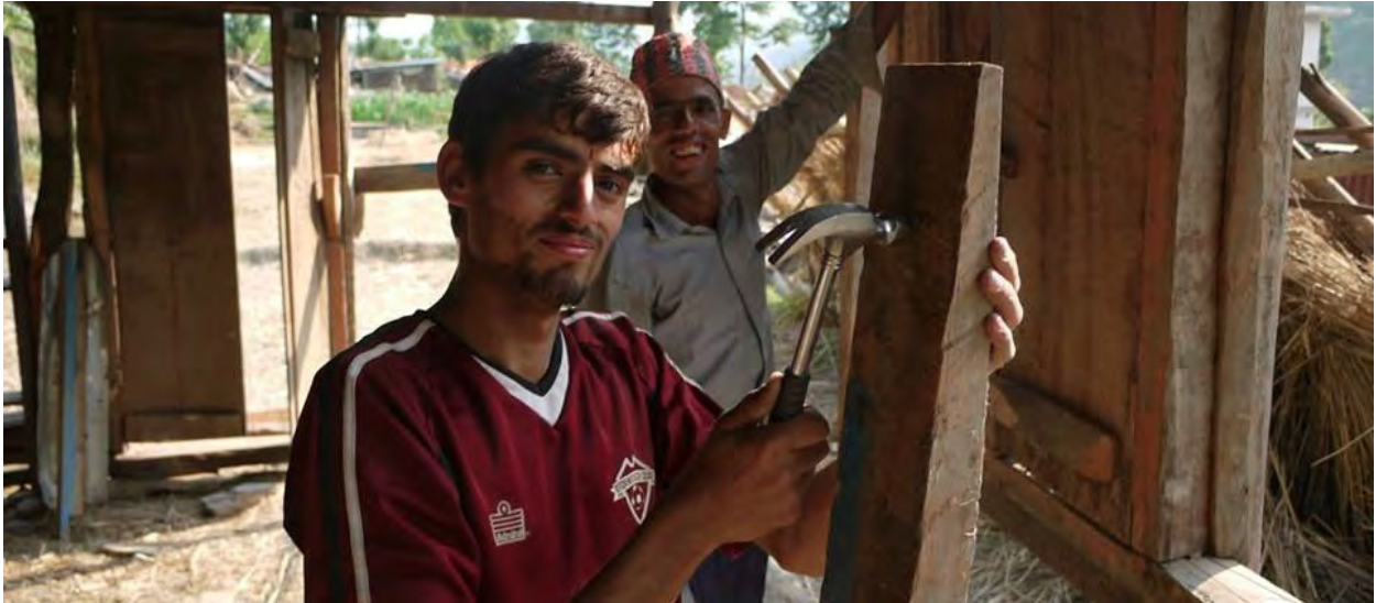
Teaching Surya Dev how to salvage local materials for reconstruction in Sindhupalchok
