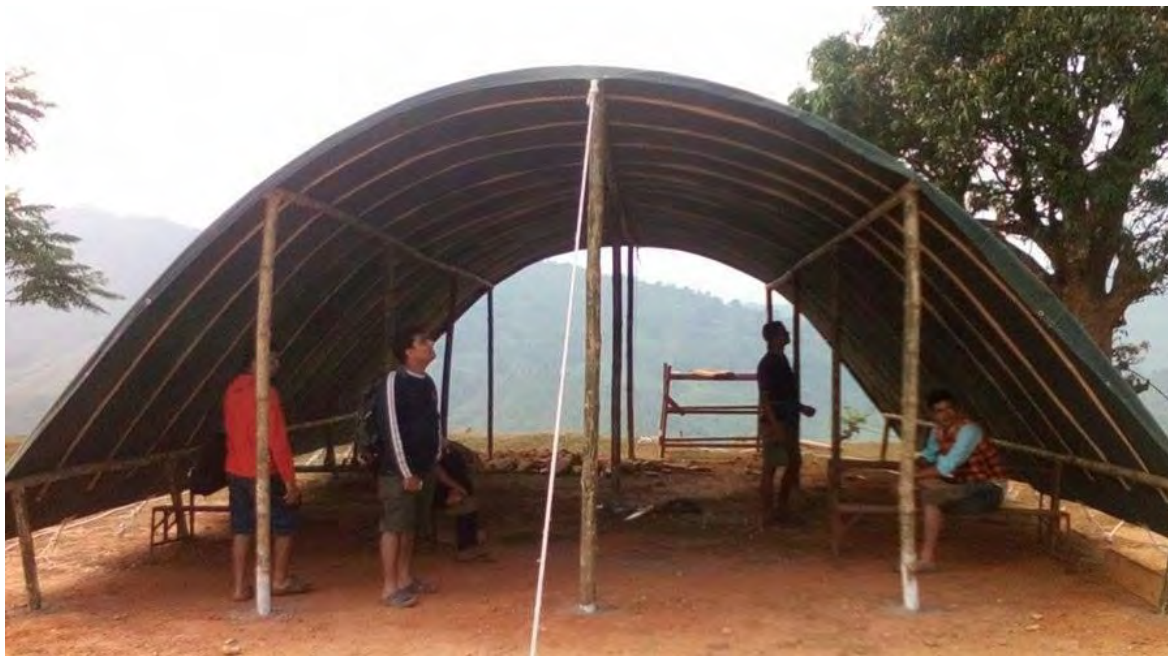
Vaulted structures are spacious and wind resistant
