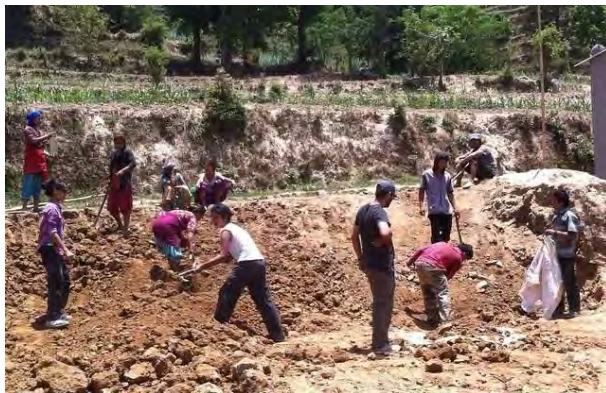
(Left: Group of residents and volunteers work together to make wide terraces for the foundation Right: Volunteers set up canvas over the foundation works)
