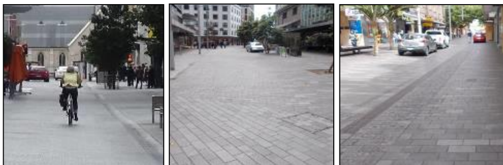
Figure 8: Insufficient 'side friction' – Federal Street, Fort Street (east), and Darby Street
