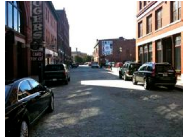
With the exception of a few “missing teeth,” the buildings surrounding Middle Street provide it with excellent spatial definition.
