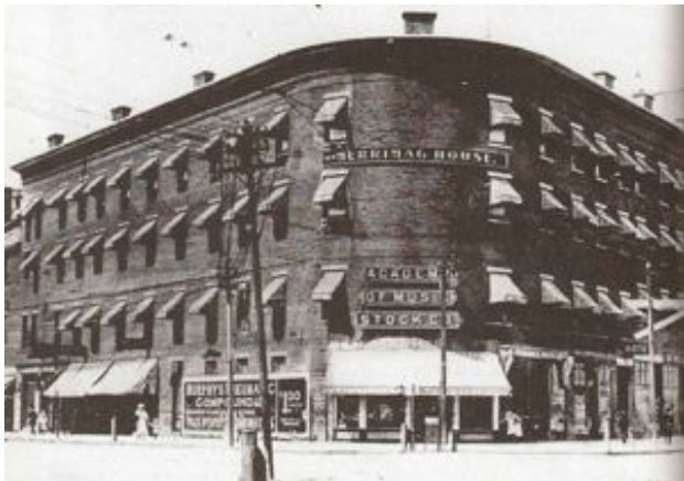
The former occupant of the Hess Station site.
