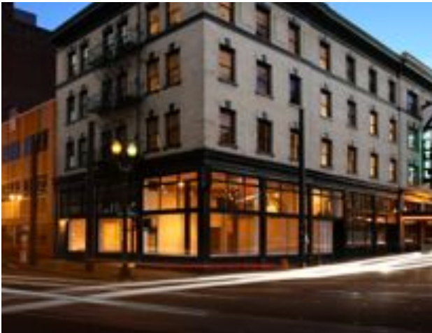
Missing in Lowell: an urban-style downtown hotel of any scale.
