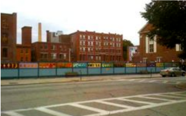
One large empty lot interrupts the healthy urban fabric of the historic core.
