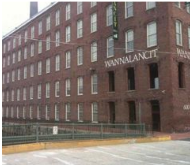
The Wannalancit Mills contain one of the largest concentrations of office space in Lowell.
