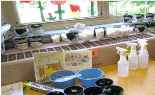
Plants and other items placed on top and in front of ventilation equipment can contribute to poor indoor air quality
