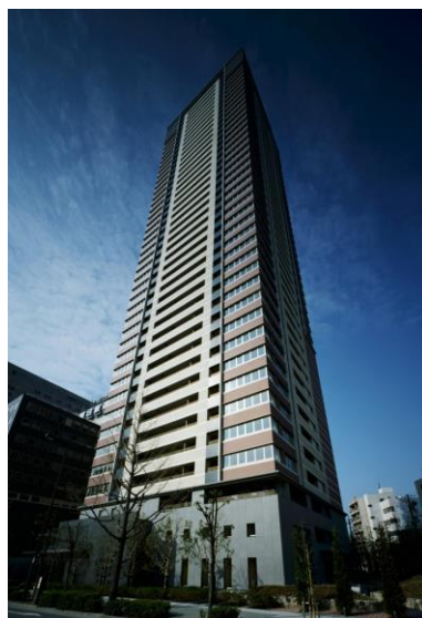
Figure 19 – Residential tower in Osaka, Japan with RFDs
