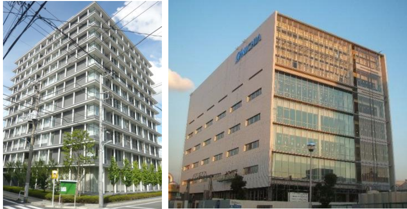
Figure 18 – (Left) 12 storey apartment building in Tokyo. (Right) 7 storey laboratory building in Yokohama
