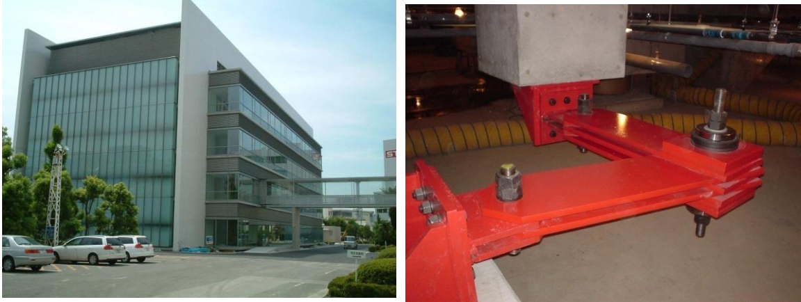
Figure 16 – a: 5 Storey Laboratory building. b: Damper installed at the base of the building
