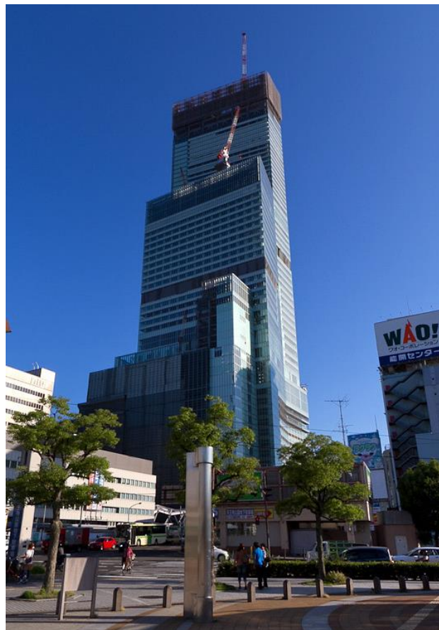
Figure 22- Abeno Harukas October 2012 (under construction)
