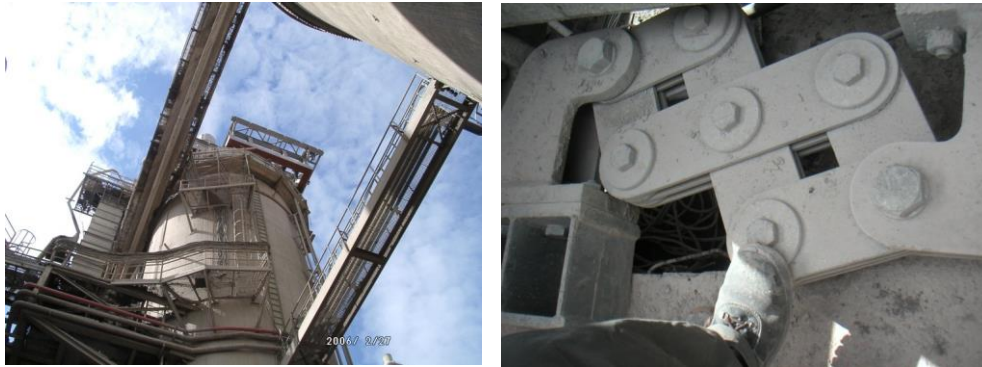
Figure 9 – Scissor Dampers in Industrial plant in Greece
