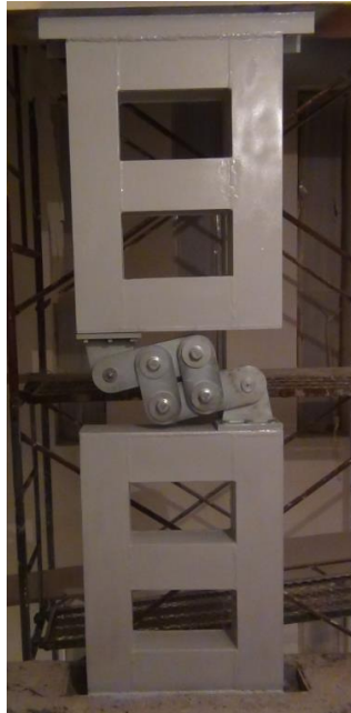
Figure 31 – Panel Damper installed in building in China
