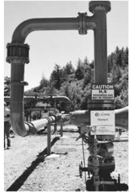
Is there a wastewater injection well near your house?
