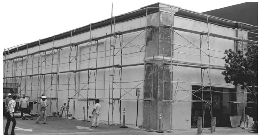
Private contractors paint over the murals. PHOTO BY MIKE RITTO
