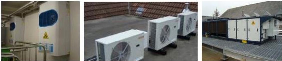
Figure 9, Examples of hydrocarbon refrigerant systems
