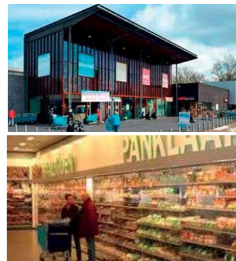
Fig. 1 Ahold Supermarket, Netherlands
