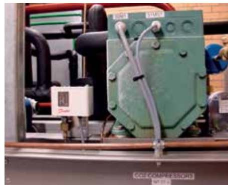
Fig. 3 CO 2 compressor in Pick'n'Pay store at Strand
