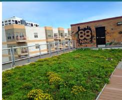
A green roof, or living roof, is a roof that is partially or completely covered with vegetation and a soil medium. Similar to a green wall, green roofs are great insulators for energy. They can also be a place of refuge for occupants of the building.
