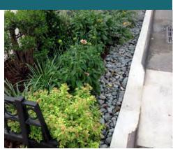
Bioswales are designed to remove pollution and settle solids from surface runoff water. They are engineered to physically and biologically treat a specified quantity of stormwater. They are not necessarily intended/designed to infiltrate stormwater and reduce peak discharge rates, but can be designed to dissipate runoff velocity and peak flow quantity. Improving stormwater quality is the primary objective with this type of GI strategy.
