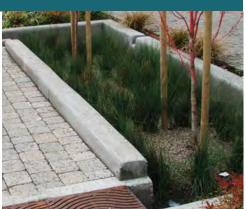
There isn't a definition specific to the term stormwater trees. The term is used to define the use, not the product. **Stormwater trees** are trees planted for the specific use of assisting in the management of stormwater. For example, trees planted in a forest are just trees. However, trees planted adjacent to a parking lot in a green space intended to manage runoff from the parking lot are stormwater trees.
