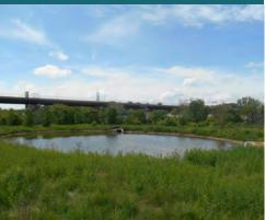
Detention/retention ponds and infiltration basins/
