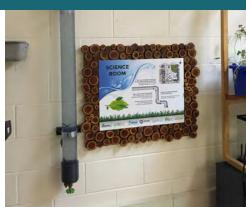
Many schools have a flat roof. Most flat roofs have internal storm drains to manage rainwater that falls onto the roof. These internal storm drains run through a series of pipes inside the building and connect to a main drain pipe. This main drain pipe eventually runs underground and connects to the sewer. Depending on your location, this might be a storm sewer or a combined (storm and sanitary) sewer.
