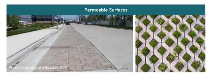
There are many types of **permeable surfaces** such as permeable concrete and asphalt, pavers and various products that offer the ability to infiltrate stormwater while providing a structurally reinforced surface.
