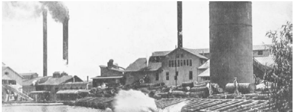
1906 view of the Crossett Company’s two original large mills. Logs hauled to the site by rail were stored in the mill pond until needed at the mill.
