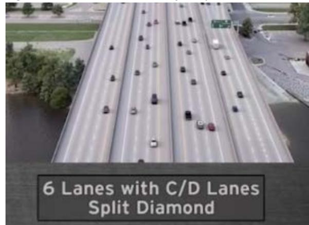
Figure 2: 12-Lane Bridge Alternative Lane Configuration
