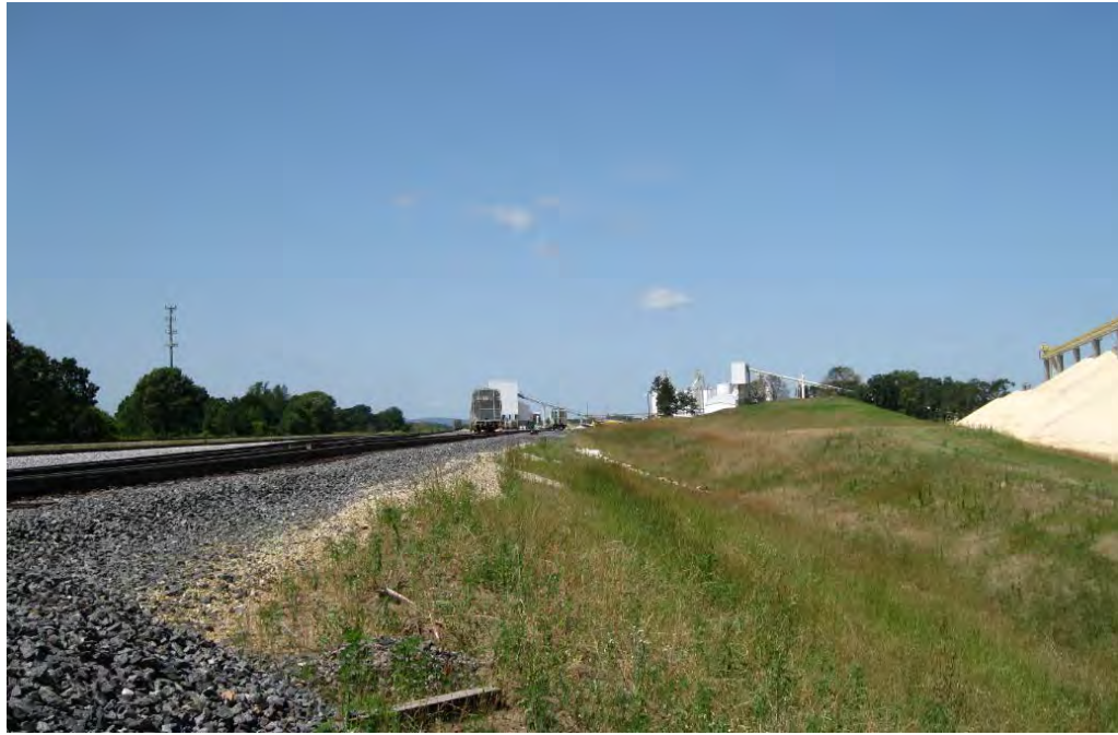
Figure 1-10 A rail siding (photo Roberta Walls, DNR)
