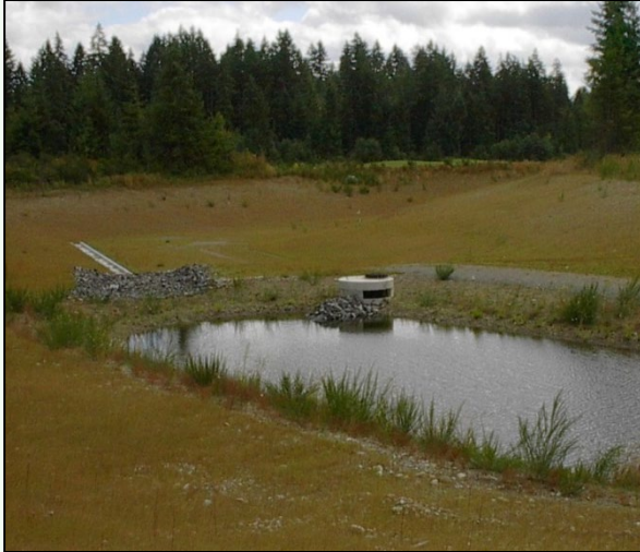
Stormwater management ponds (dry or wet)
