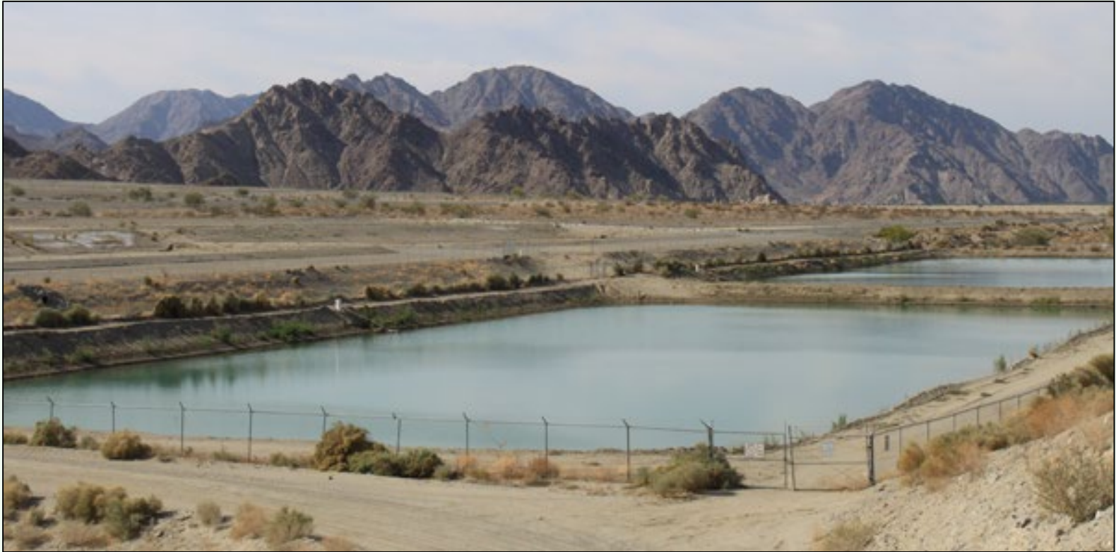
Groundwater recharge basins
