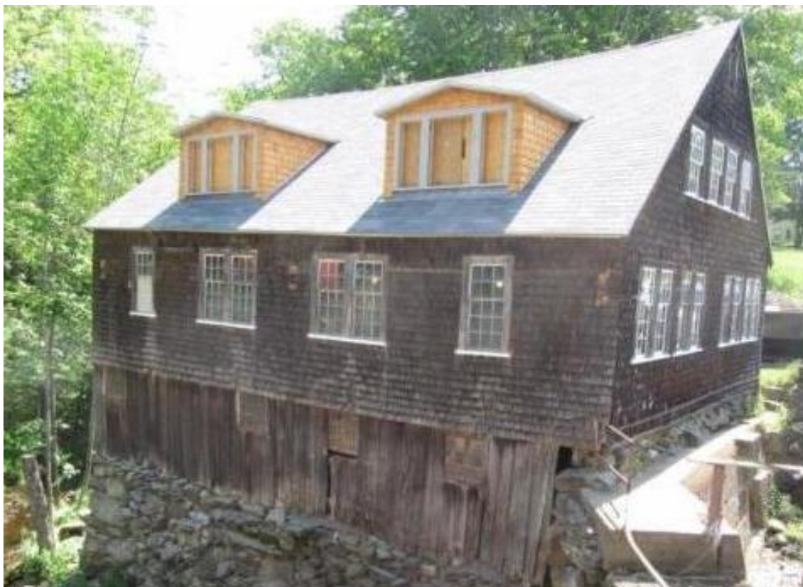
Two of the three new dormers and new roof.
