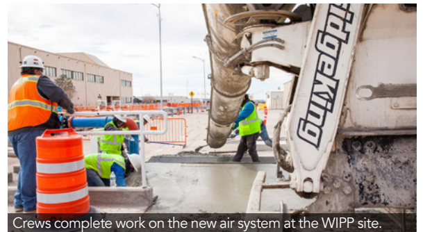
Crews complete work on the new air system at the WIPP site.
