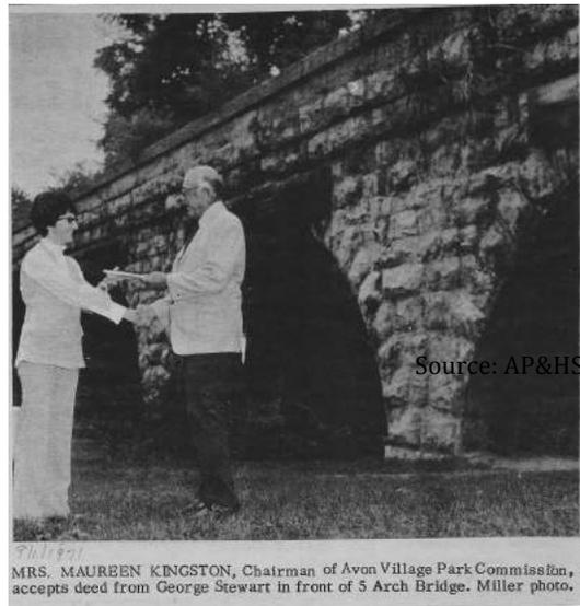
In 1985, an engineering study by Bero Associates of Rochester viewed the structure as in fair shape, but it was suffering from water penetrating through the railroad bed. The report noted that rainwater was dissolving the mortar holding the stones together, thus weakening the structure. The recommendation to restore the structure suggested removing the trees, brush and debris and installing a roof to create a water disposal system as well as repairing the mortar joints.
