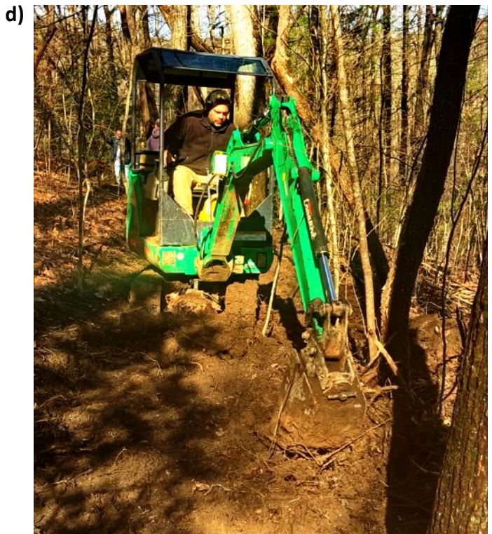
Figure 5. Photos illustrating: a) the flat camping area near the Hawk Mountain Shelter, in comparison to b) and c), sustainable side-hill campsites constructed in sloping terrain; d) mechanized construction of the side-hill sites; and e) GATC volunteers at work.
