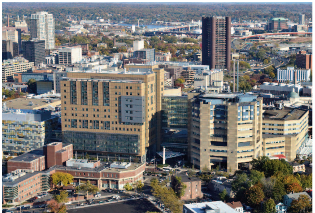
Aerial view of the Smilow Cancer Hospital, the large building in the left half of the photograph. Founded in 2009 as part of Yale-New Haven Hospital, the state-of-the-art cancer treatment center, named for philanthropist Joel R. Smilow (B.A. 1954), typifies the expansion and modernization of Yale's medical campus and of its research and clinical capabilities.
