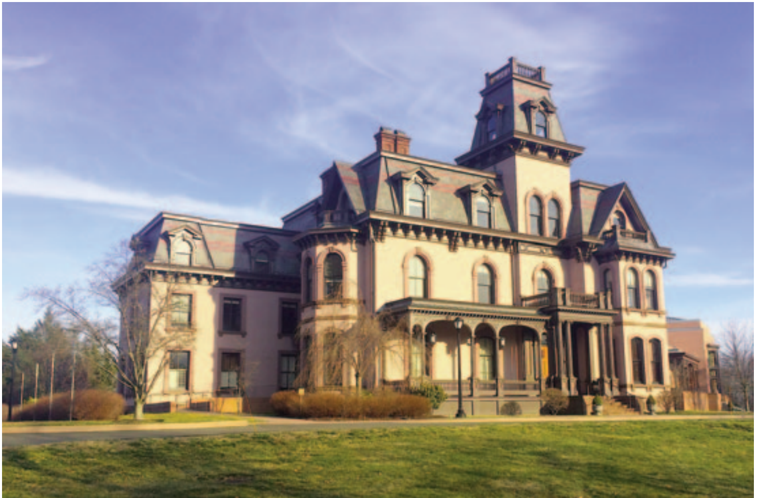
Betts House, on upper Prospect Street, houses administrative offices.
