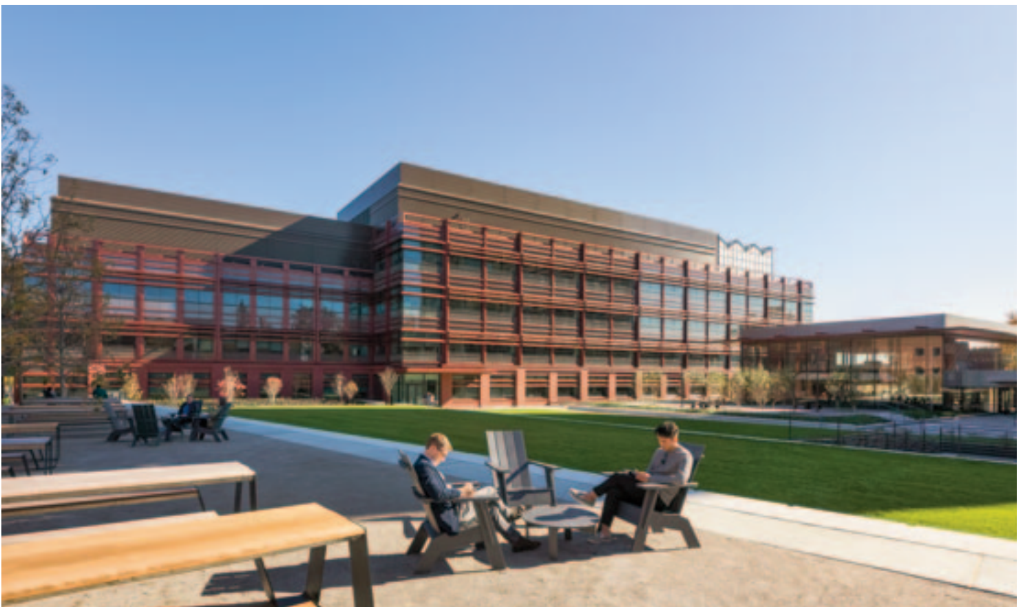
The new Yale Science Building, with 280,300 square feet of laboratory space for biology and related disciplines, opened in 2019.
