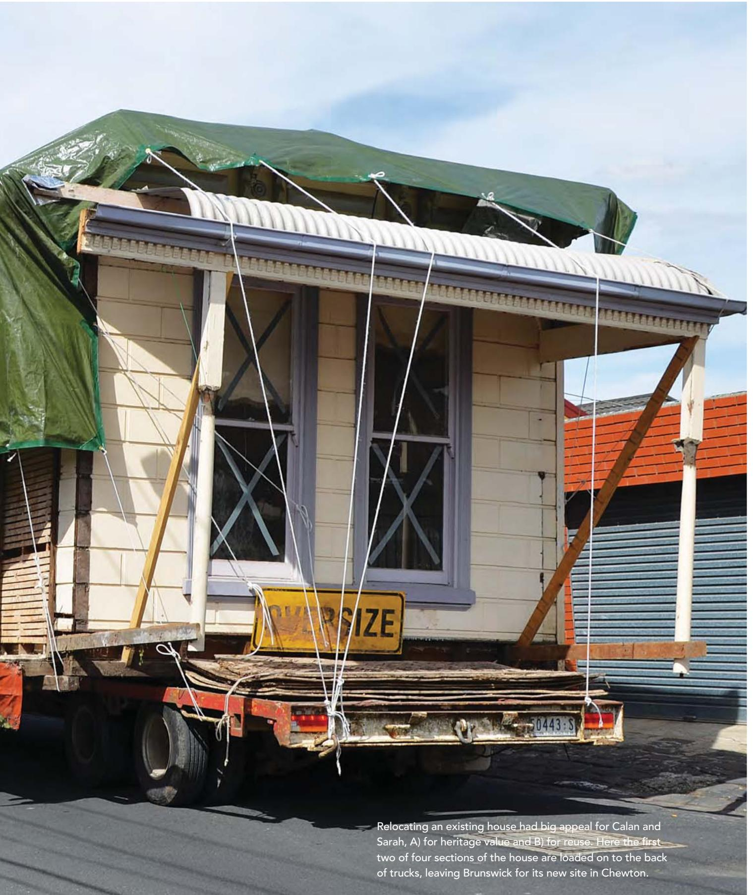
Relocating an existing house had big appeal for Calan and Sarah, A) for heritage value and B) for reuse. Here the first two of four sections of the house are loaded on to the back of trucks, leaving Brunswick for its new site in Chewton.
