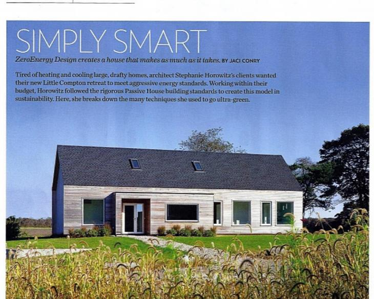
• BAN THE DRAFT The best return on a minimal investment is airtight construction, Horowitz says. To achieve this for her clients, she filled the home's 11-inch-thick walls with a medium-density spray-foam insulation. Because the foam runs continuously from the foundation's edge to the roof, drafty spots are virtually eliminated, resulting in a house that is two to three times more insulated than the building code requires.
