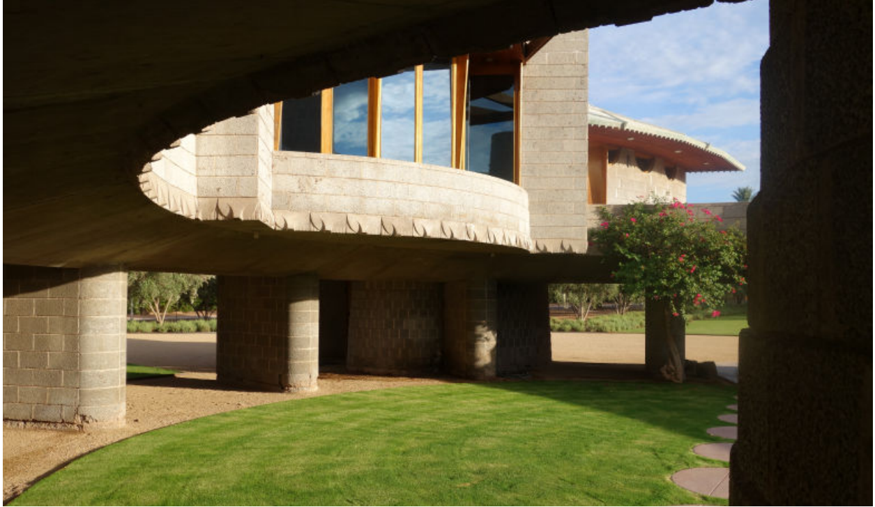
Interior of the courtyard; note the decorative cast block at the level of the floor slab. Frank Lloyd Wright never shied away from ornament. The block pattern is reminiscent of the “Textile Block” used at the Arizona Biltmore and in several Los Angeles area houses. Photo courtesy of OAI.
