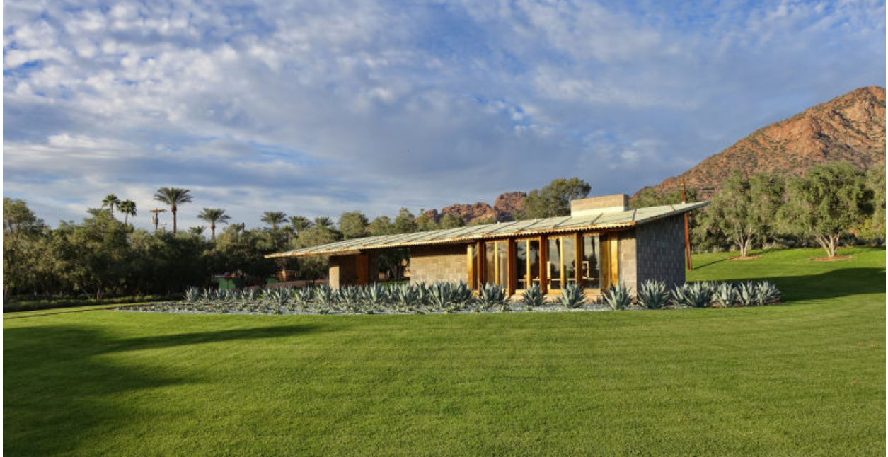
Guesthouse seen from south. Note the continuous bank of windows with roof overhang at right for passive solar gain; roof is a simple shed form sloping south with metal roof similar to main house. The sloped design was intended to create a line of sight up Camelback Mountain. Photo courtesy of OAI.
