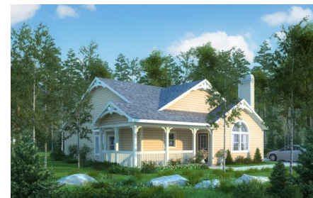
Figure 2b: Example of a properly finished corner lot.
