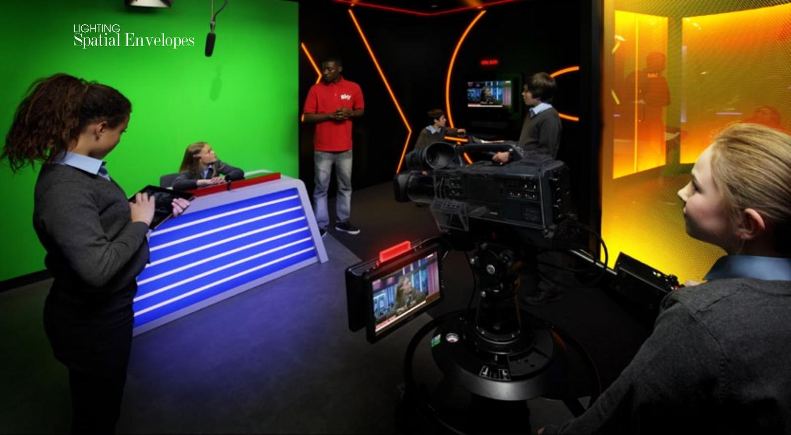
The central core production space consists of a suspended light box, which is backlit by strings of RGB LED, which is DMX-controlled over several channels, this enables the lighting to morph through varying hues of colour, linked in with the Sky corporate spectrum colour scheme.
