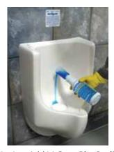
3. Just Add It! Pour BlueSeal® directly into trap insert or cartridge.
