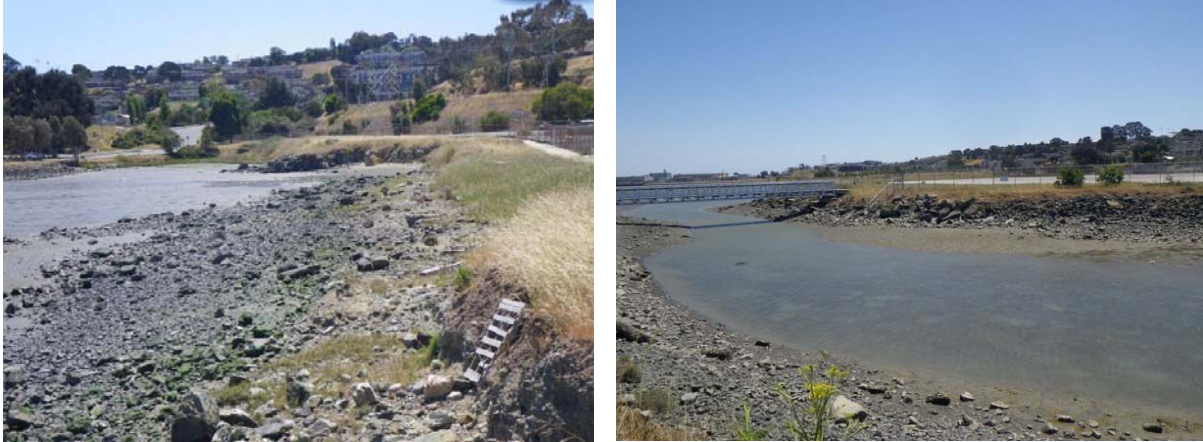
Figure 13: Typical Conditions Along Reach PGE-R1, R2 (left) and Reach PGE-R3, R4 (right)
