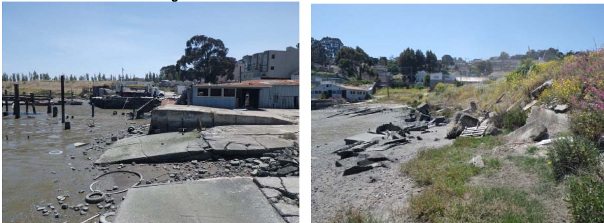
Figure 8: Typical Conditions Along Reach 900-R1 (left) and Reach 900-R2 (right)
