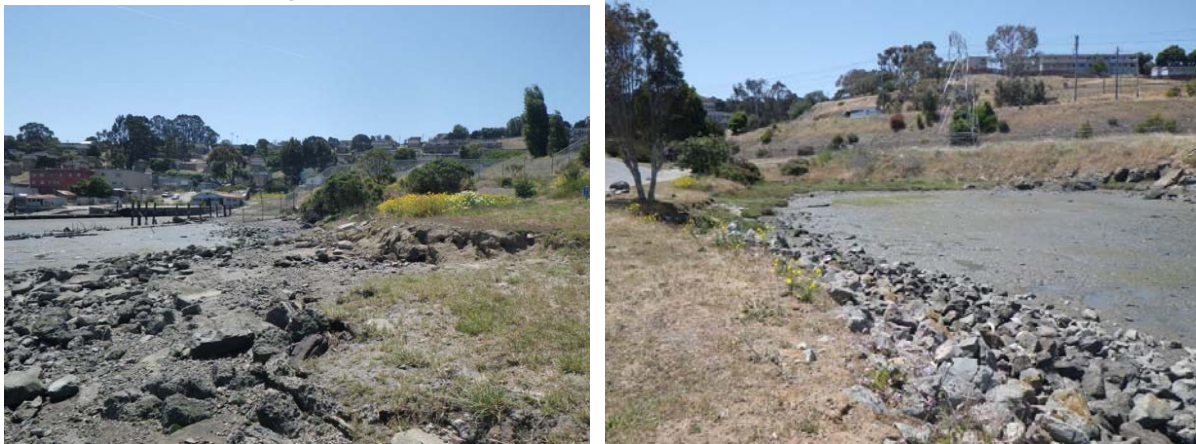
Figure 10: Typical Conditions Along Reach IBSP-R1 (left) and Reach IBSP-R4 (right)
