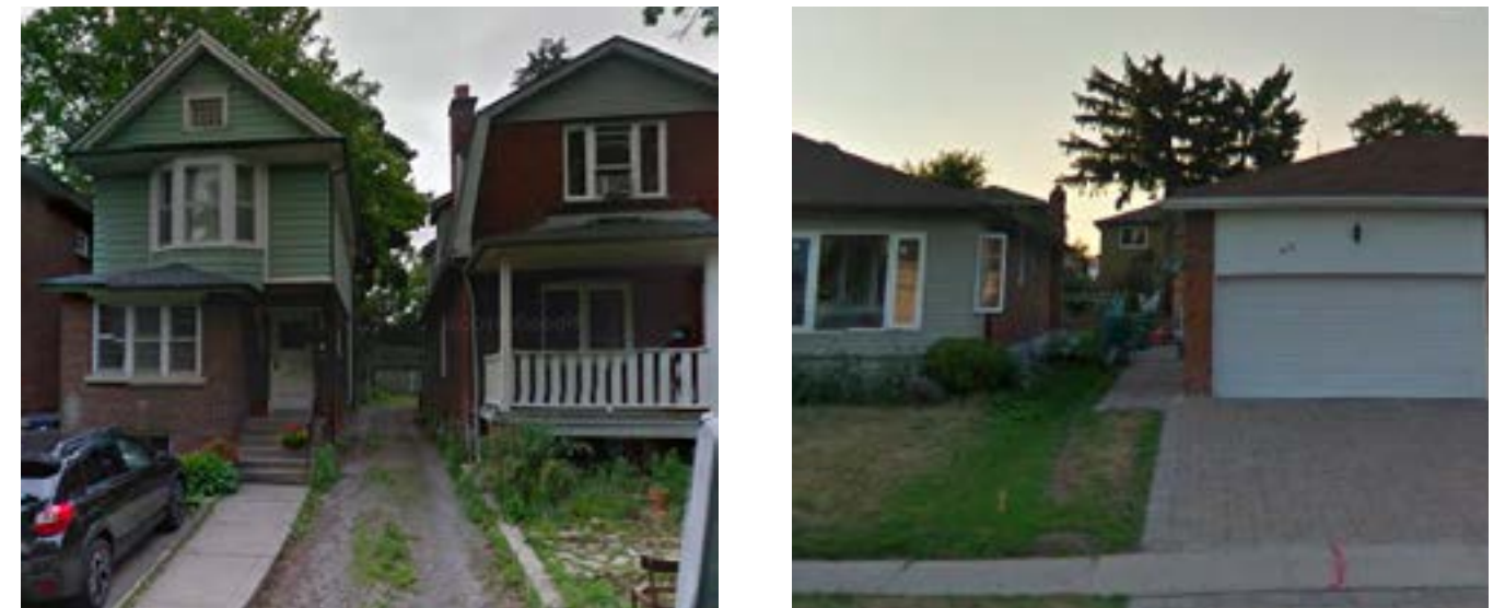
Figure 8: Depicting examples of minimum 4 foot accessways between houses in Wards 18 (on the left) and 41 (right).
