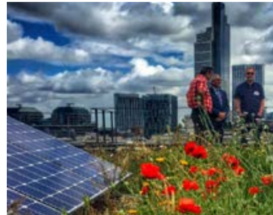
Bio-solar roofs manage stormwater and collect solar power.
