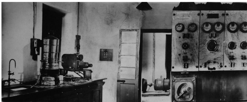
Figure 7. The control panel and curator's room, with a view into the room housing the motor-generator. Image courtesy of the Government Museum, Chennai.
