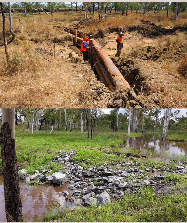
TOP: Leaky weir being constructed at Mt Pleasant Learning Hub, September 2019. BOTTOM: Leaky weir after rains, February 2020.
