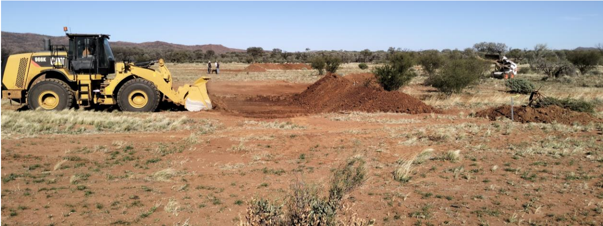
Figure 2. Constructing earth banks in Central Australia
