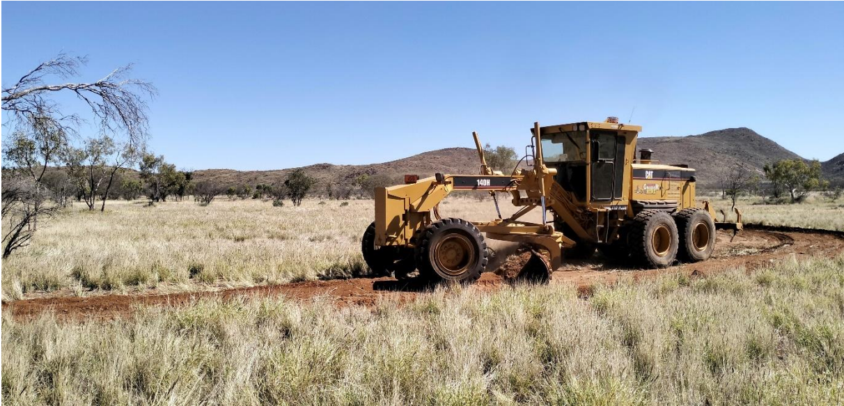
Figure 51 Completing the primary sill on contour 3 at Narwietooma.
