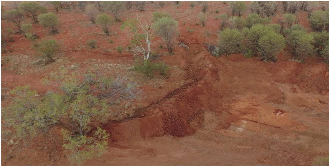
Figure 55 Earth flow around in-stream structure at Glen Helen lower floodplain just after construction (November 2022). Note near end toe anchored against tree and curvature of structure (flow direction right to left).
