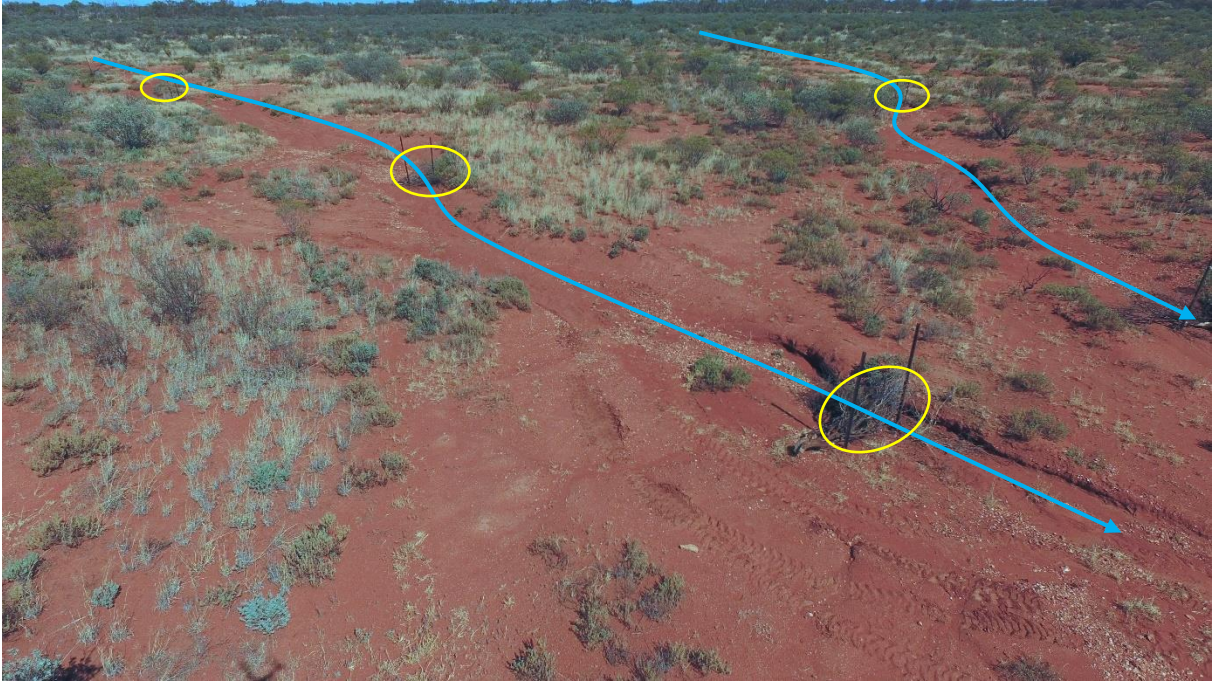
Figure 45 A series of small stake and brush weirs on multiple gullies above the road.
