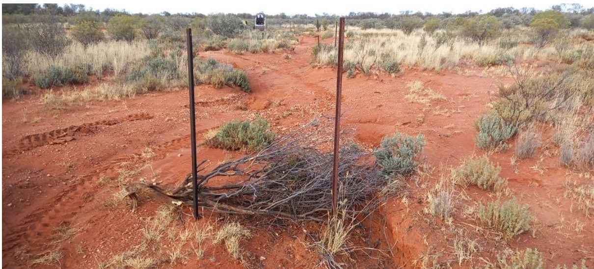
Figure 29 Example of a stake and brush weir in-stream structure with brush placed on the upstream side. Sediment and organic material will become trapped and continue to accumulate.
