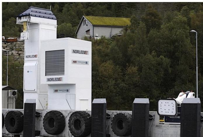
Once the vessel is being supported by shore power, its power converters will begin charging the battery arrays at a controllable rate intended to ensure that the energy deficit from the last transit is recovered
