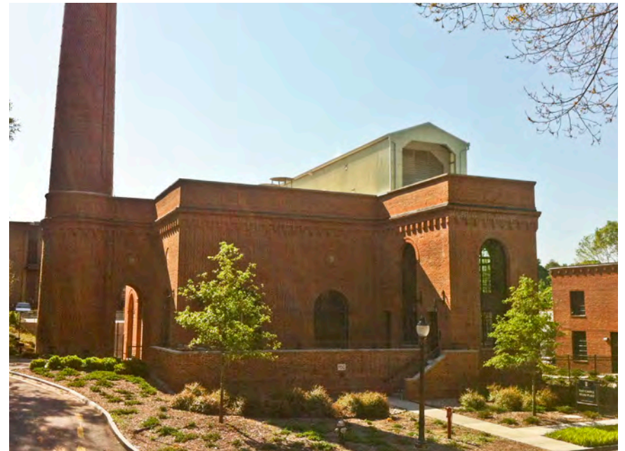
Recently renovated steam plant in the proposed Arts District.
