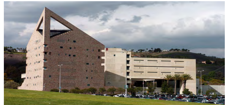
Soon-to-be-demolished 17 year old Cal Polytechnic Pamona tower in a park.
