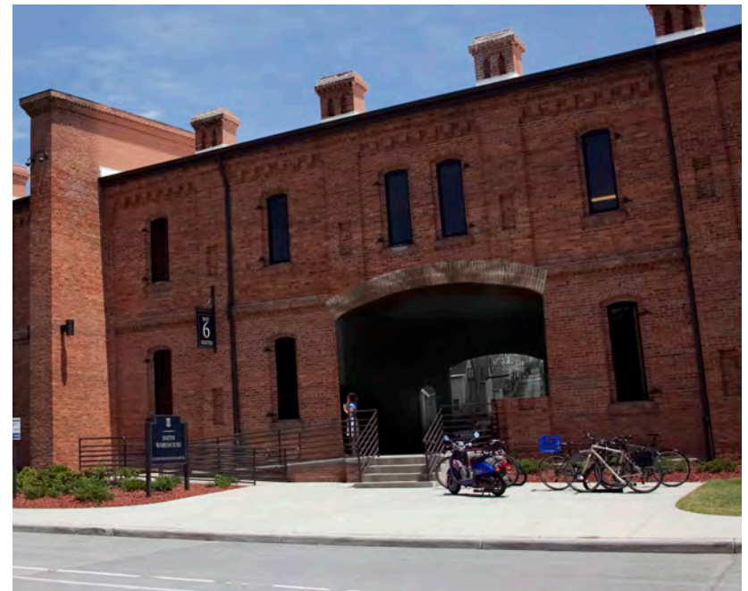
New ground level passageway through building to residential row houses to the South. The location is marked by an asterisk (*) in the plan to the left.
