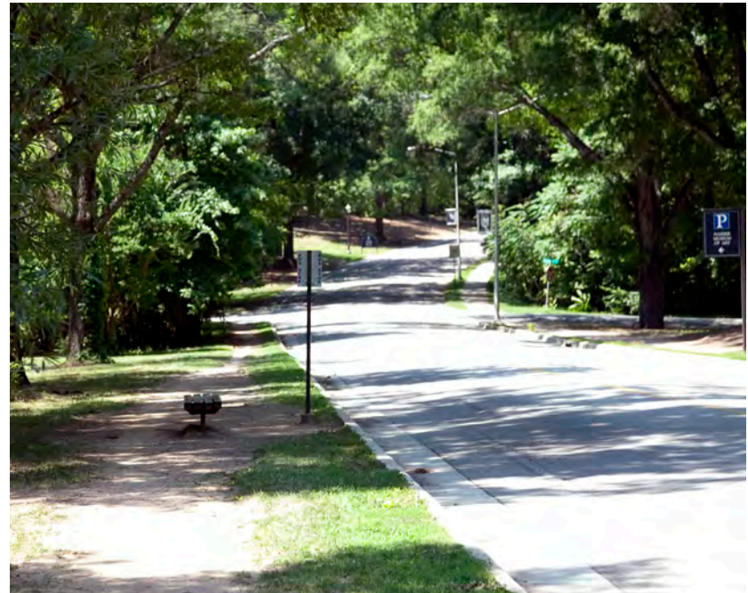
Existing stretch along Campus Drive.
