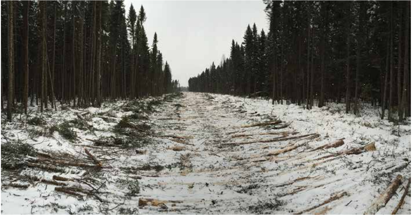
Rieger's crew built several skid trails like this one, using tamarack to fortify the road, then built trails off either side to access the black spruce.
