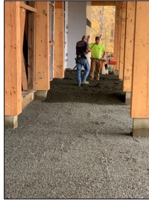
Laying subsoil for final surface of veranda
