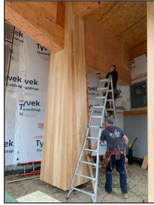
Finishing columns with cypress
